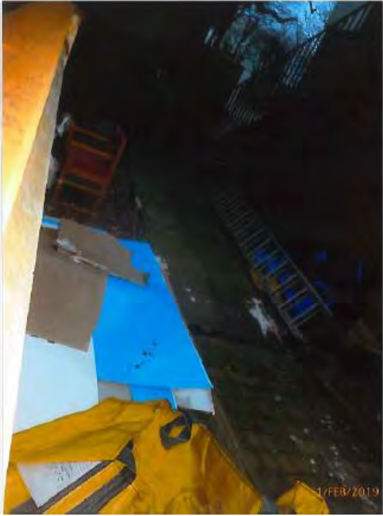
Physical damage and emergency exit
